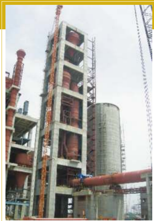
Ariyalur project in progress - Pre Heater
