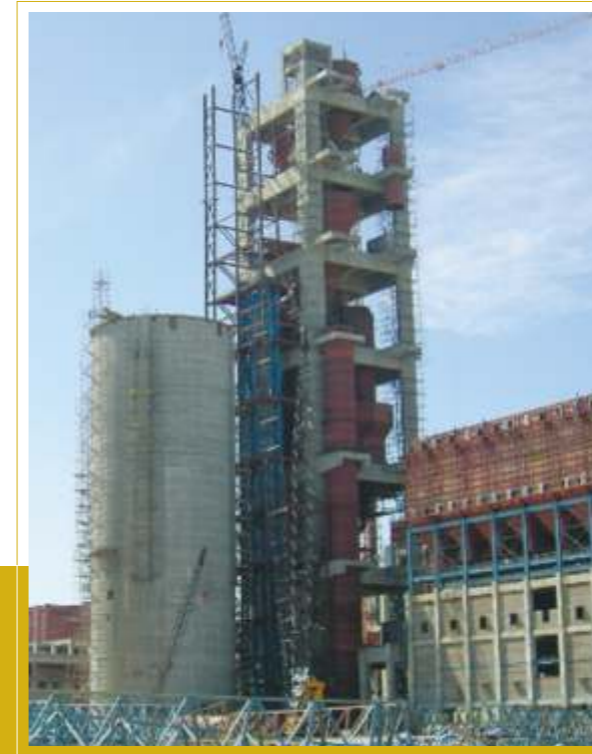
Ariyalur project in progress - Blending Silo, Preheater and Bag House
