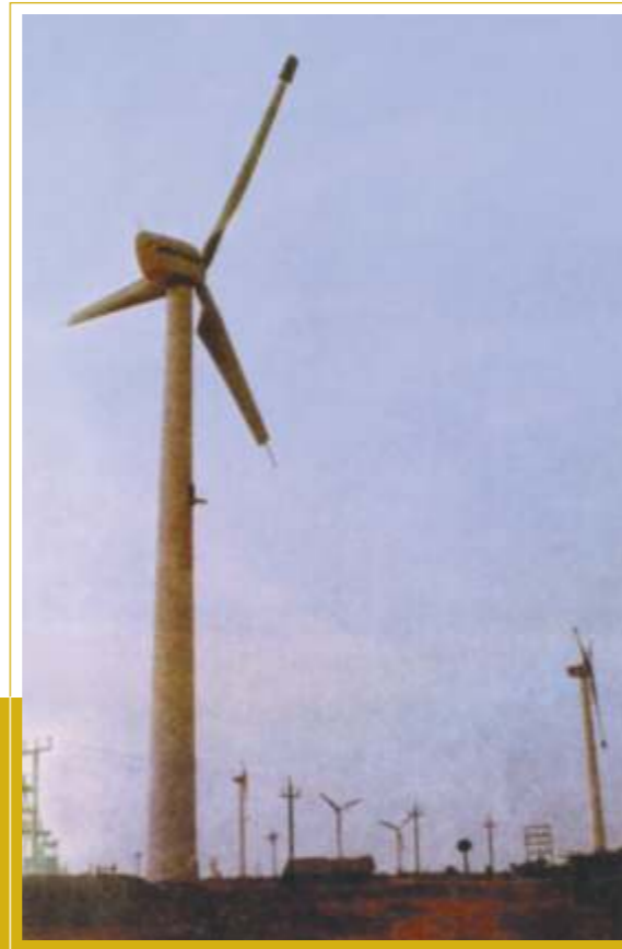
The new Wind farm at Coimbatore District
