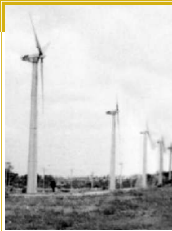
The windfarm at Muppandal, Kanyakumari District
